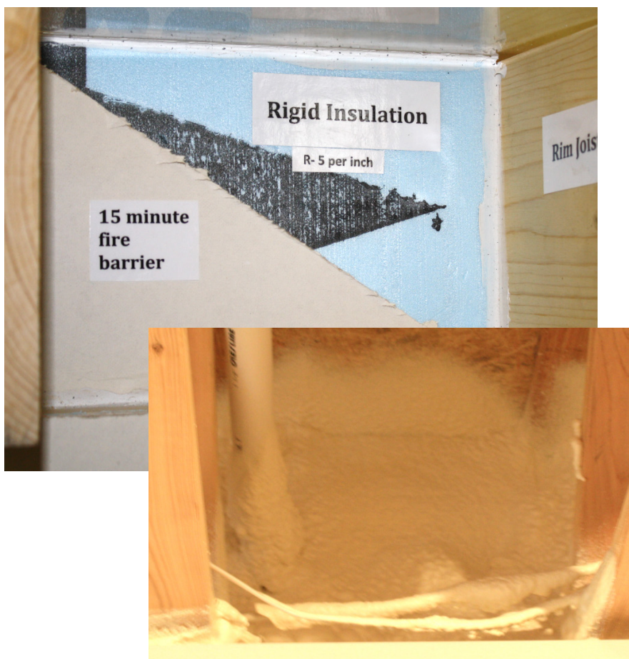
Figure 7. Insulating the rim joist and sealing air leaks with rigid insulation or expanding spray foam. Insulation needs to be covered with a 15-minute fire barrier.
