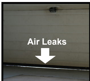
Figure 4. Air leaks resulting in wasted heat. (Carl Pedersen, NDSU)
