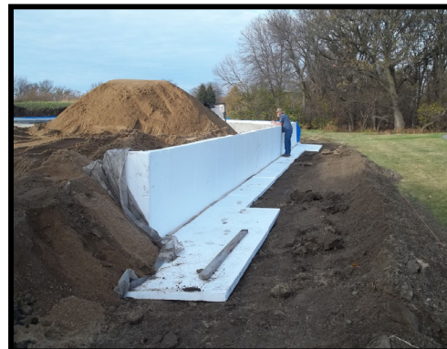
Figure 7. Frost-protected shallow footing foundation for heated slab. (Larry Mayer, Solution Design Inc.)
