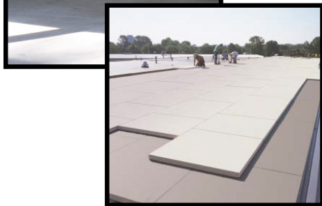
Figure 5. Continuous insulation on roof deck. (U.S. Department of Energy)
