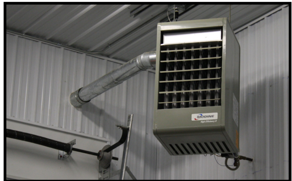
Figure 1. Forced-air propane furnace. (Carl Pedersen, NDSU)
