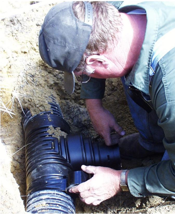
One or more special control structures, or the pumped outlet itself, may be used to control the drainage system. Control structures utilize stop-logs or baffles to set the desired water table elevation at the location of the structure; a pumped outlet may be turned off to create the same effect.
