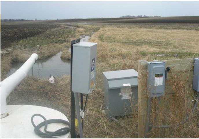
Pumped outlets increase the initial investment and operation/maintenance costs of the tile drainage system but may be economically feasible in many situations. A pumped outlet station includes a sump, pump, discharge pipe and usually an electric control panel. Important design features include the storage volume of the sump and capacity (flow rate) of the pump.
